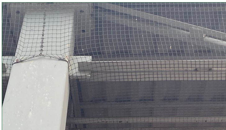
Figure 3. Bird netting on a building.
